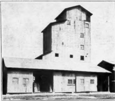
Mixing Mill House
